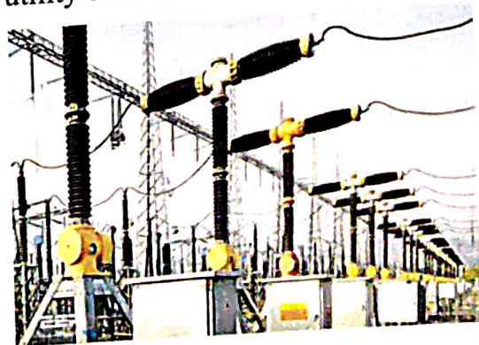
Fig. 3.2 High voltage switch gear installation
