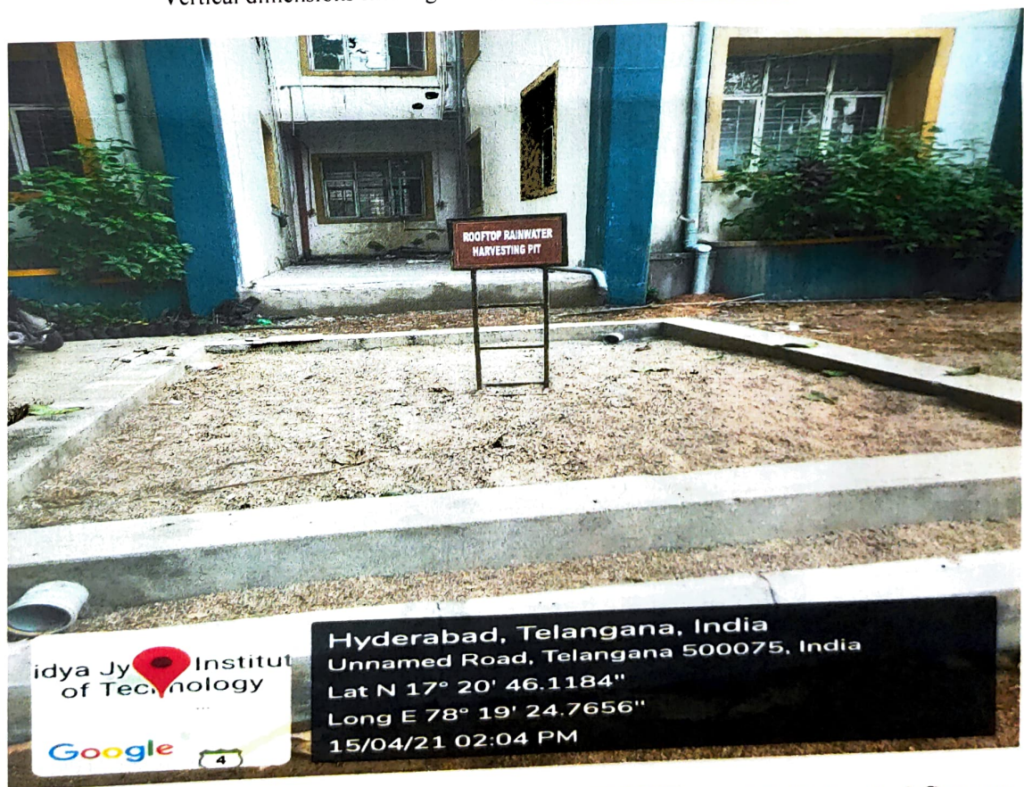
Roof top Rain Water Harvesting Pit of Size 10ft X 10ft X 8ft in VJIT, Hyderabad Campus
